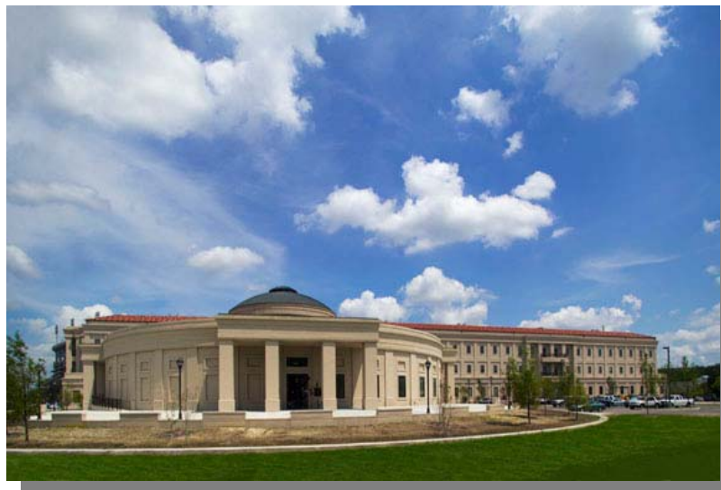
Energy, Coast, & Environment Building, 2003-present
