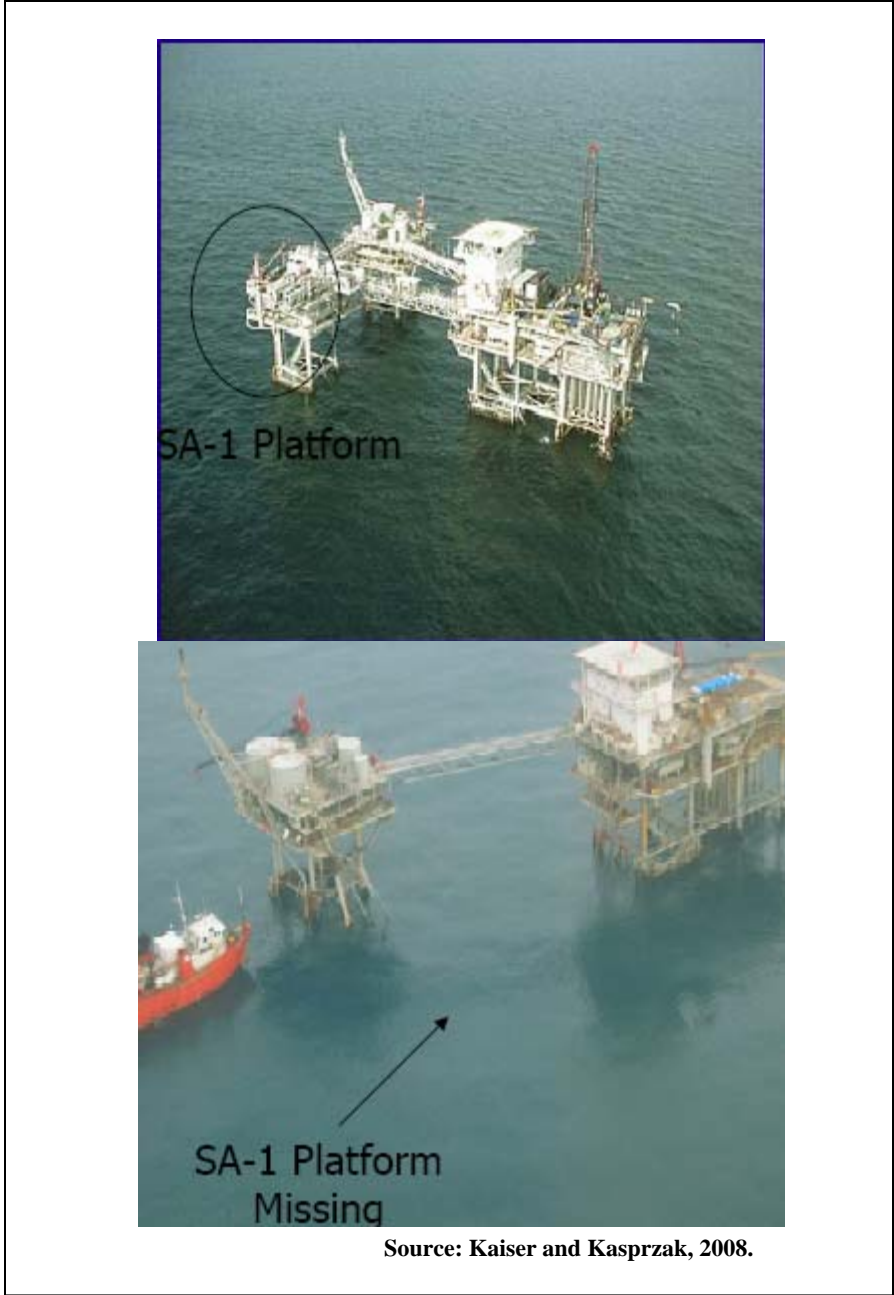
Figure D.3. Before and After - Devon Energy's SA-1 Platform Destroyed at South Marsh 128.
