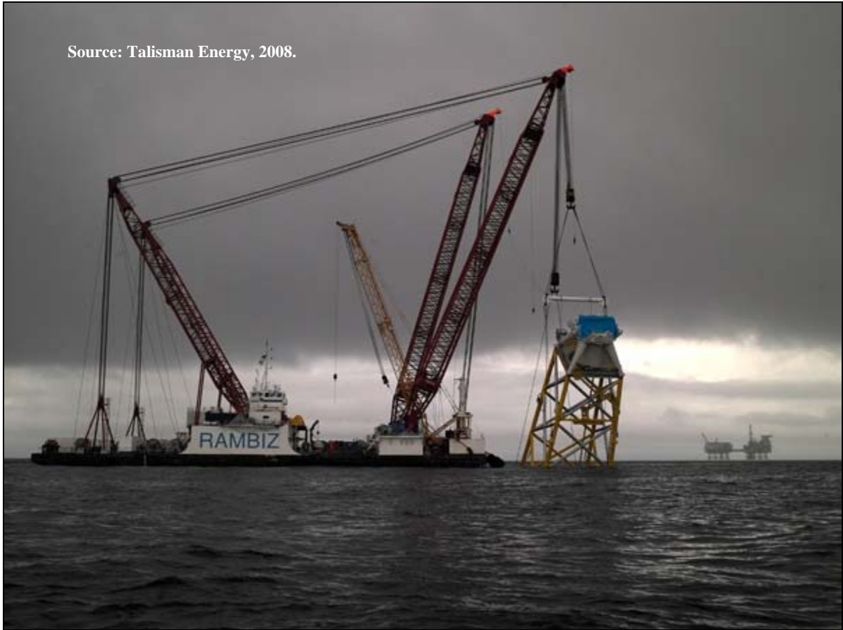
Figure G.15. Sinking of a Jacketed Foundation for the Beatrice Project.
