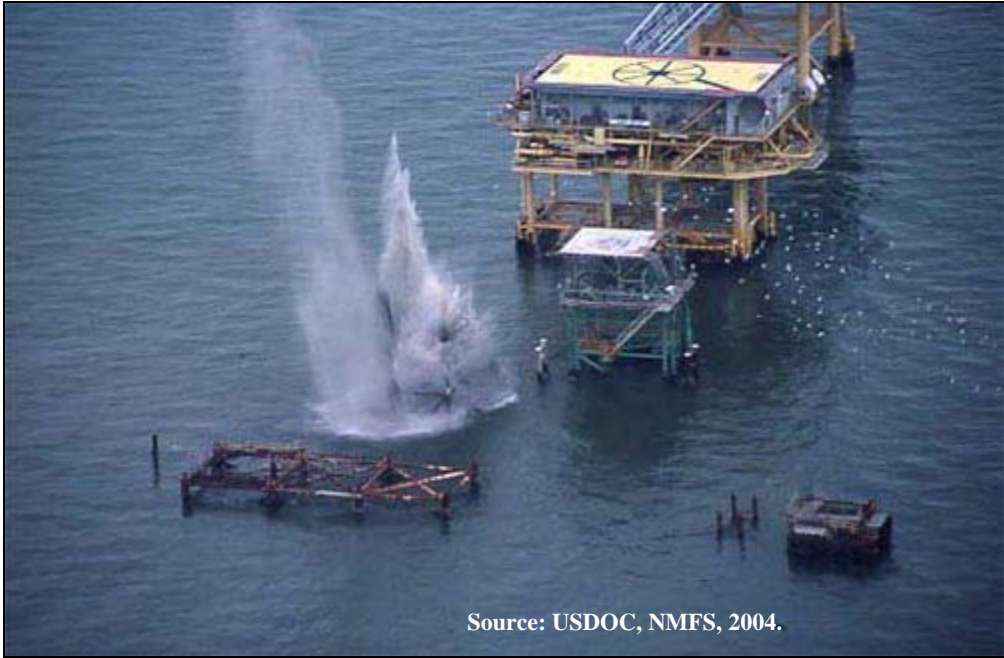
Figure A.11. Aerial View of Job Site during Blast and Detonation.
