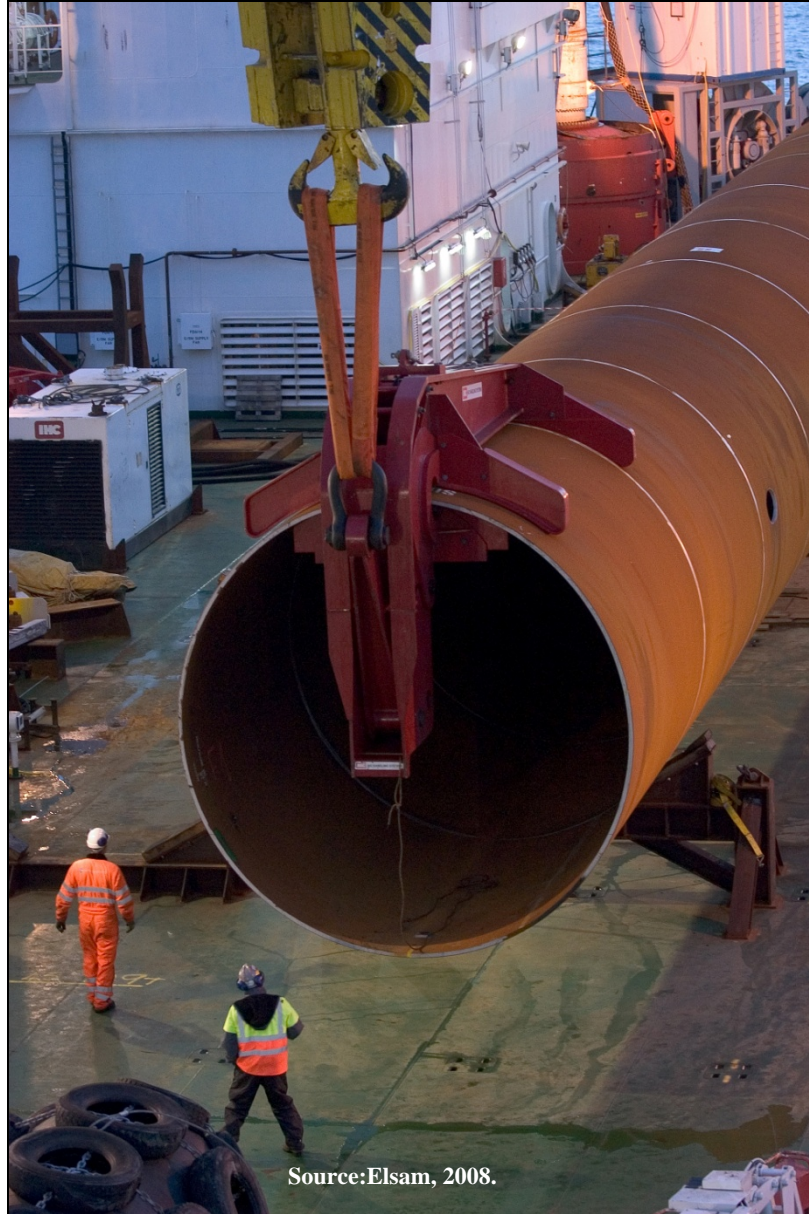
Figure G.19. Monopile for Use at Kentish Flats.
