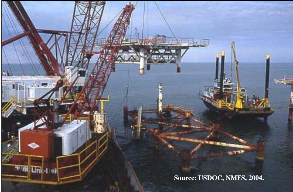
Figure A.9. Derrick Barge Arrives On-Site and Removes the Deck Module.
