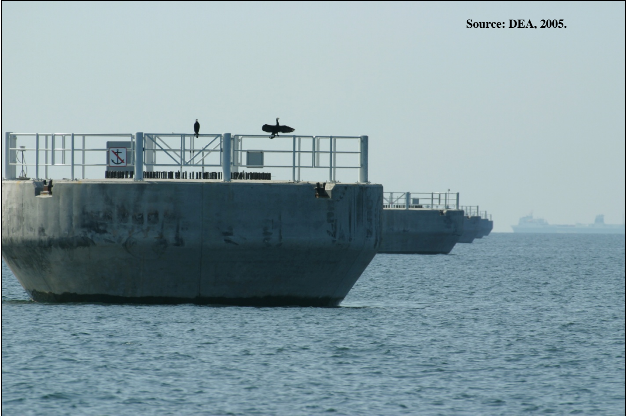
Figure G.18. Gravity Foundations at Nysted.
