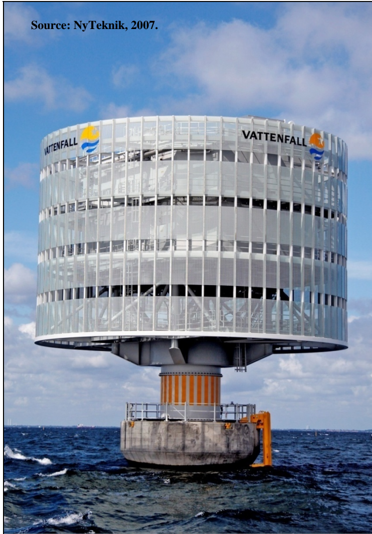
Figure G.11. Electrical Service Platform at Lillgrund.
