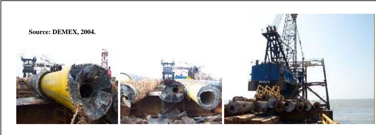
Figure A.12. Severed Piles and Conductors Loaded onto Derrick Barge.
