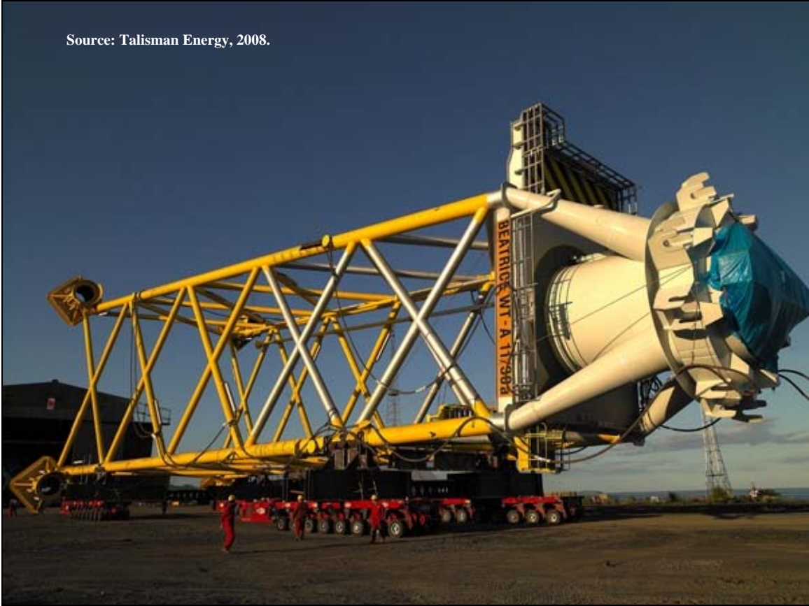
Figure G.14. Beatrice Jacket Foundation. Note People in Foreground for Scale.
