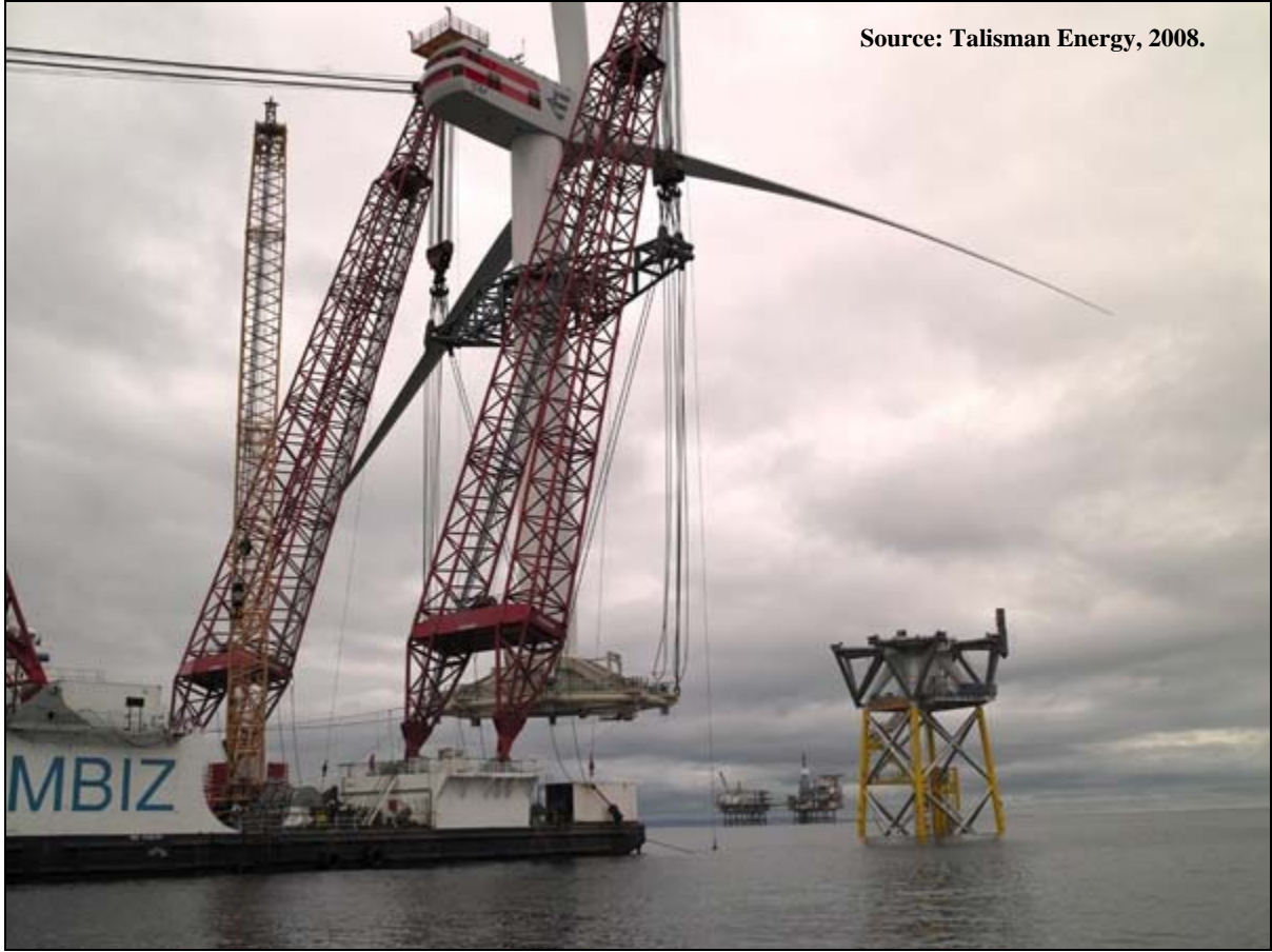
Figure G.16. Lifting of the Beatrice Turbine and Foundation.
