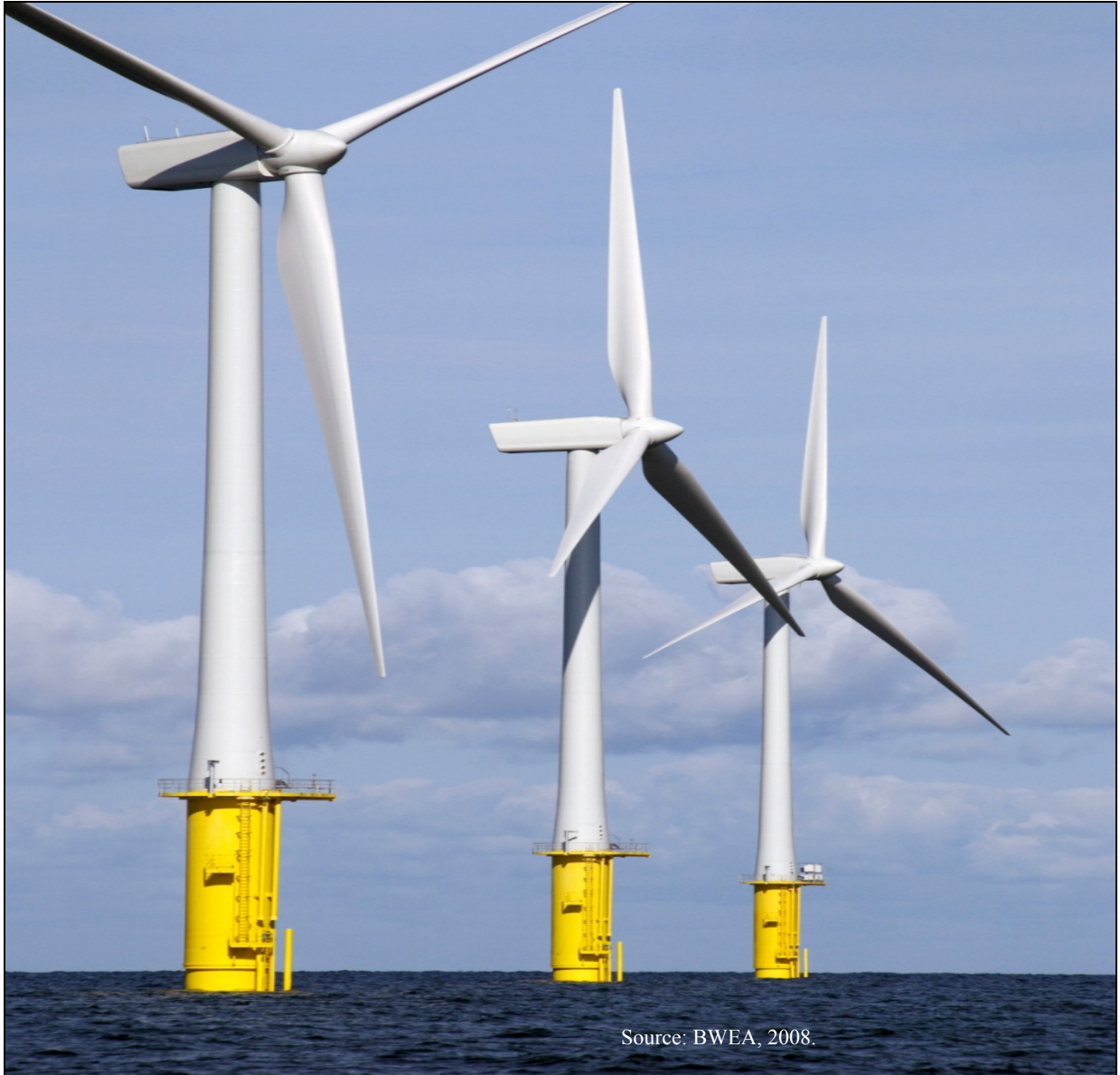
Figure G.8b. Row of Turbines at North Hoyle Showing Transition Piece Painted Yellow for Navigational Purposes.
